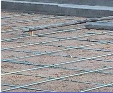
4MAX™ Composite Rebar is a high-strength composite reinforcing bar from MST-BAR®, engineered for concrete flatwork. 4MAX™ Composite Rebar replaces steel rebar and welded wire mesh in flatwork, providing centuries of serviceability to your reinforced concrete.
